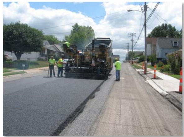
Paving operations on Hoffmeister Avenue
