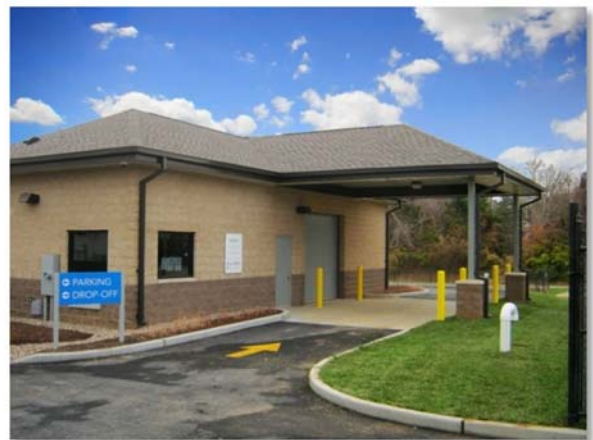
South County Hazardous Household Waste Disposal Facility
