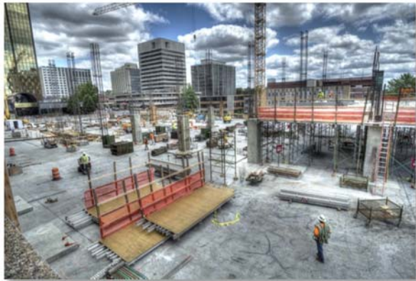
Construction of the new County Courts Building
